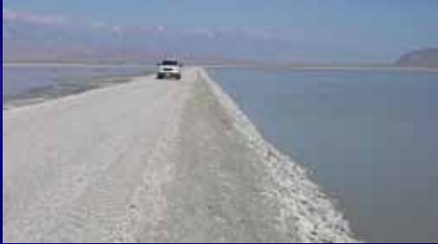
Containment berms and ponds
